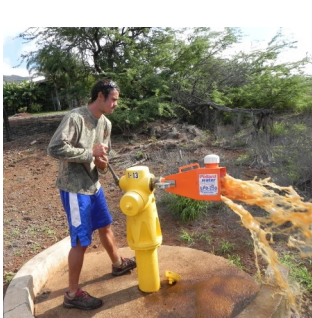
Troy setting up diffuser to Hydrant and then showing why we do Annual flushing of KPHA-Water System
