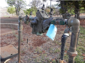
All lots with water in Kawela Plantation Homeowners Assn. have backflow preventers (BFPs). These BFPs are tested and repaired annually.
